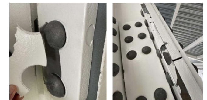
Brittle fracture of the intumescent PFP coating
